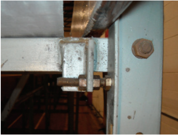
A unique feature found on Wayne bleachers are these manual horizontal and vertical adjustment screws. These are not available in new bleacher systems.
