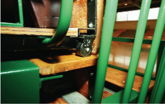
Continuous support wheel in closed position.
