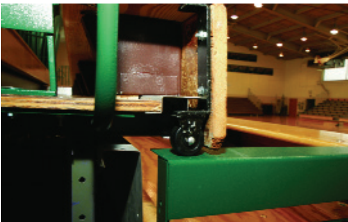
Continuous support wheel in full open position.
