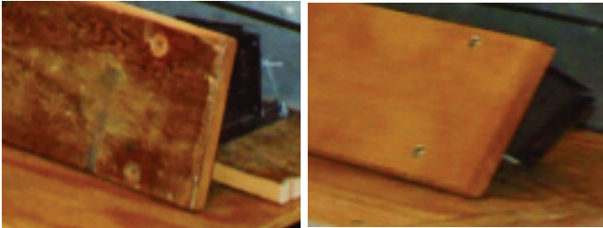
Fifty-year-old Fir seats before refinishing (at left). After planing, sanding and edging, the same lumber (at right) looks new again. Re-installed with new hardware, this seat is ready for another fifty years.
