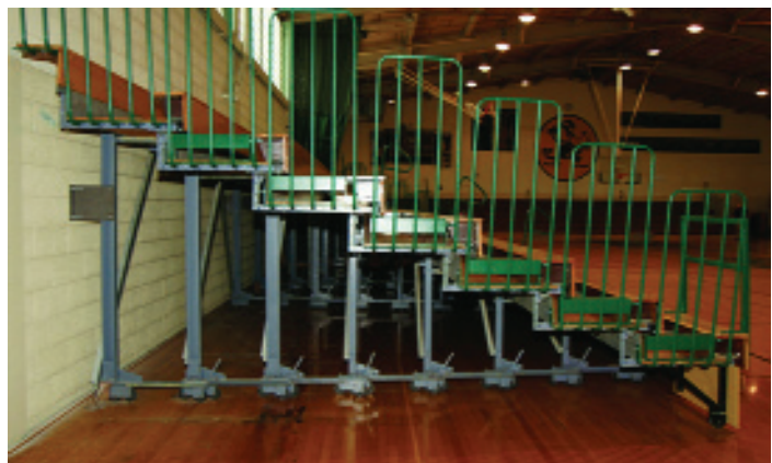
End view shows vertical support columns.
