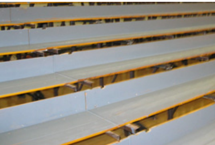
Heelboards and footboards are painted a contrasting color of wear-resistant enamel. Note flush fit (no gaps) between sections.
