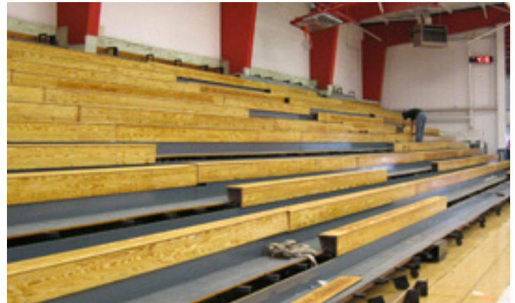
What a difference. after the original wood is planed, edged, sanded and sealed. It's hard to believe it's the same wood!
