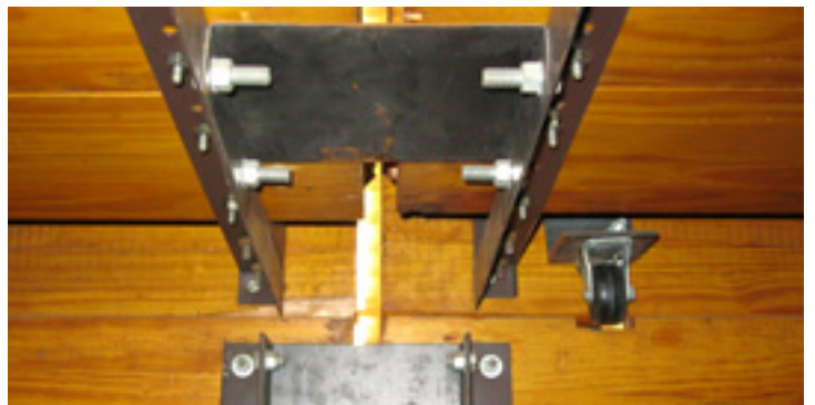
Original row ties shown here do NOT close the gap between sections, which requires that the bleachers be unbolted from the wall and pushed together to fit flush. Note wheel on footboard does NOT provide continuous support like the Century Design® system does.
