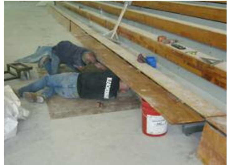
Preparing mount for new motorized drives to be installed.
