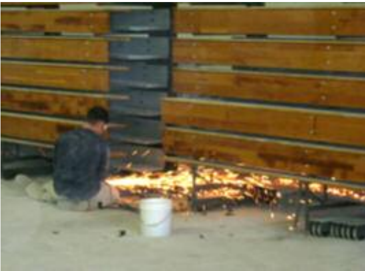
Bleacherman crew member prepping understructure for new nosebeam assembly.
