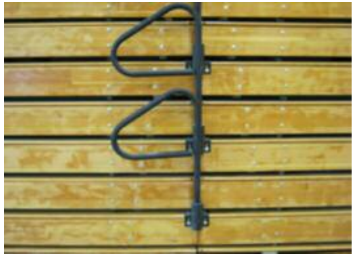
Refinished Fir lumber shows the natural color variations that are typical for this material.
