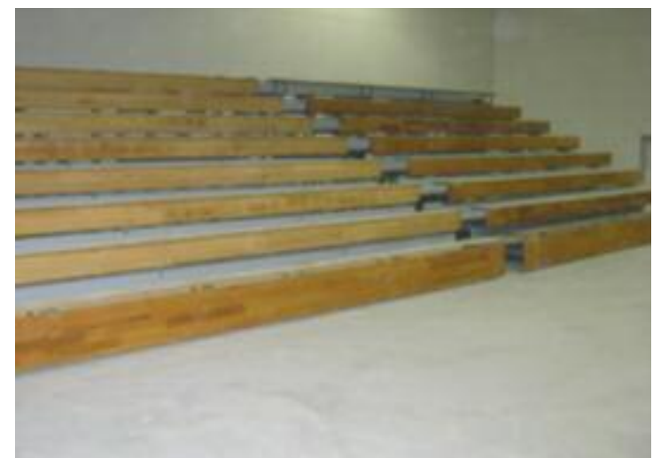
Bleacher section in the foreground is ready for stain application, to match bleachers in background.
