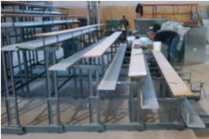
In this picture, the understructure has been reconditioned and painted.
