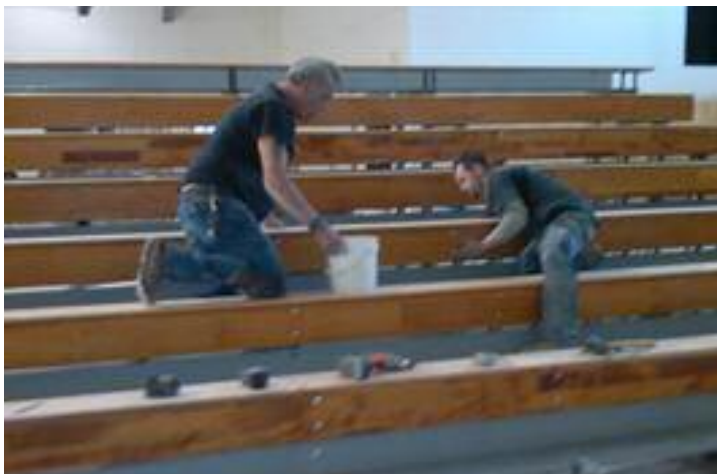
Crew members installing risers.
