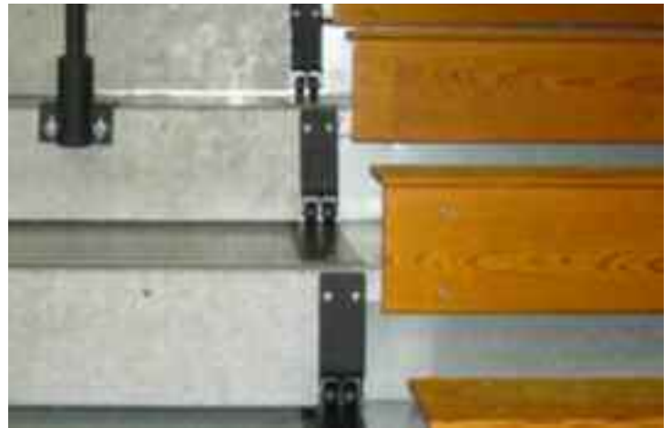
Century Design® was also installed at the aisles. A two-wheel design on one side of the aisle is used here due to the sagging issues, instead of the more common one-wheel system, to assure long-term trouble-free use.
