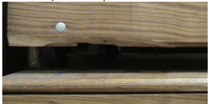
Another broken board. It will be replaced by a new board from the Bleacherman's inventory of wood, using the same species (Southern Yellow Pine) and stained to match. Our wood shop can manufacture any type or size of board needed for your bleachers: Pine, Fir, Mahogany, solid, finger-jointed, or laminated. Click here for more info.
