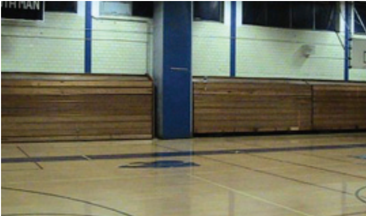
Original bleachers in closed position – No end safety rails, no aisles or ADA wheelchair spaces.
