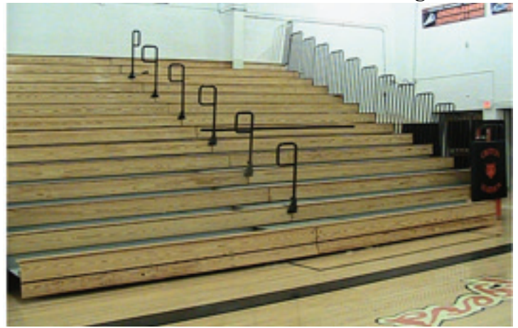
P-rail removed from where it was incorrectly installed in the first row
