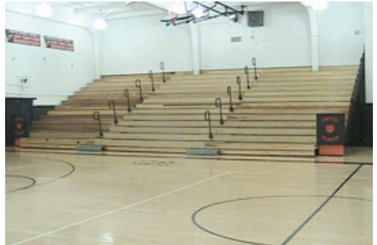
Now the bleachers have the aisles and P-rails in the correct position, second row end safety rails added, wheelchair cut-outs added. Bleachers were adjusted to provide an additional 18 inches of space from the "out-of-bounds" line to the leading edge of the first row. This space was 30 inches, now it is 48 inches.
