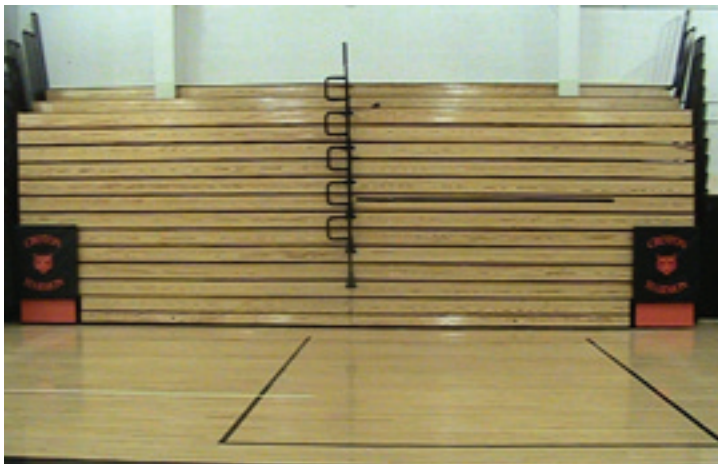
Bleacher section in closed position. Note even row spacing, now that the Century Design® no-sag system has been installed.
