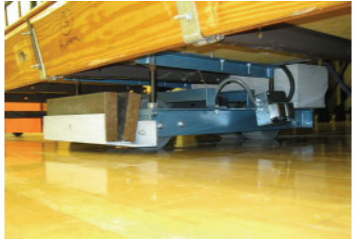
The Bleacherman installed a front counter weight so the motor drives would operate correctly, with no lifting. This engineering feat is called "common sense."
