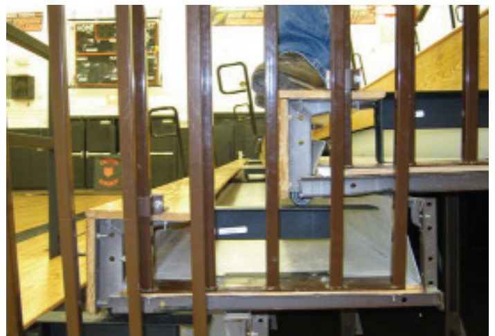
End view of third and fourth row in partial open position, showing the Century Design ® no-sag system. Note wheel on seat level "runner" supporting the live load on the row above.
