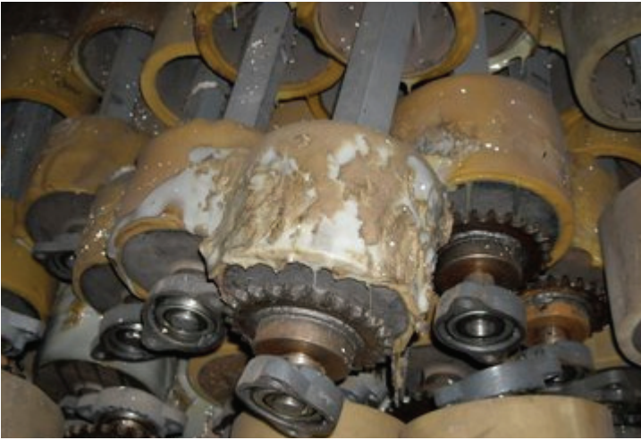
Delaminated drive rollers removed from bleacher drive units. Synthetic covers on steel rollers are decomposing and delaminating.
