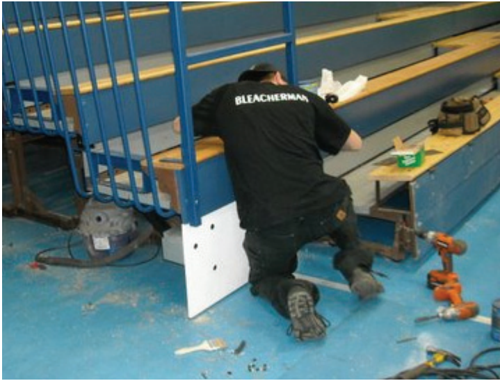
Bleacherman worker installing an ADA “cutout” to accommodate wheelchair seating.
