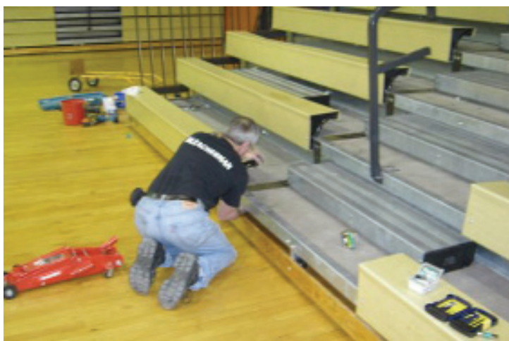
The Century Design® system that provides support at the aisles is a foot-level configuration -- the wheel rides on a runner installed on the footboard.
