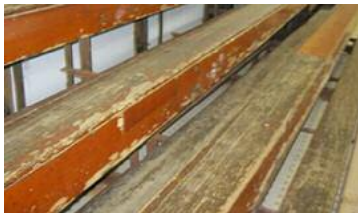
Original five row high telescopic bleachers show the effects of a high-humidity environment and years of heavy use.
