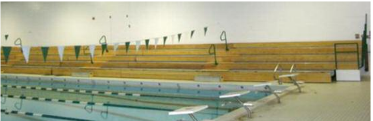
Another view of the completed bleachers. Note that the riser boards are three-piece laminated boards, which show the color variation this is normal in this material.
