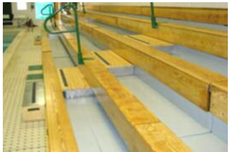
Completed bleachers with demountable first step, non-skid on intermediate steps, contrasting color footboards, etc.
