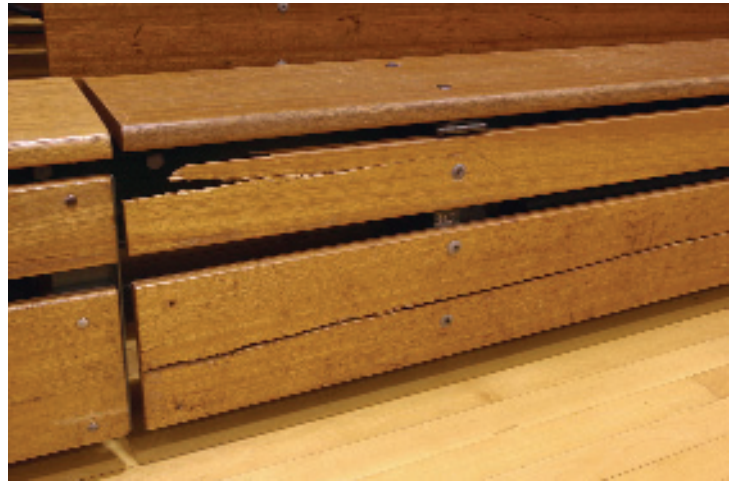
Original wood seats and risers were replaced by plastic seat modules.
