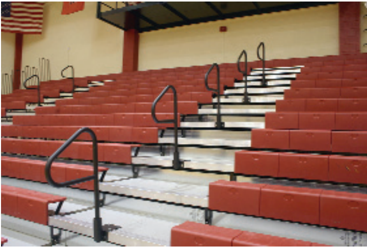
Heelboard was recycled from original bleachers and painted to match new plywood deck system
