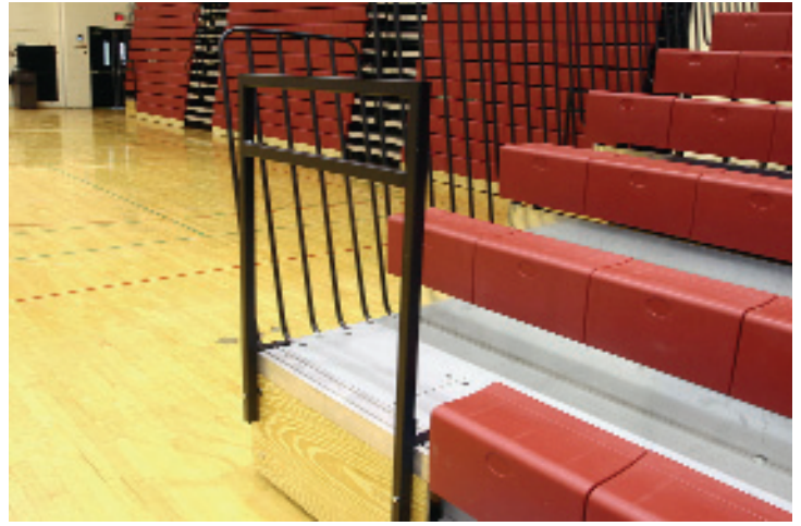
ADA wheelchair cut-out for handicapped seating.
