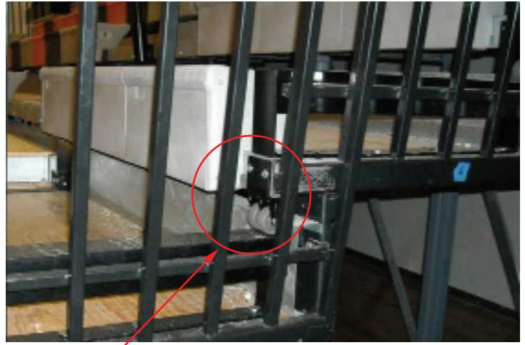
The Century Design® system is shown here, at the ends of the bleachers. This reinforces the understructure and eliminates the damage caused by climbing.
