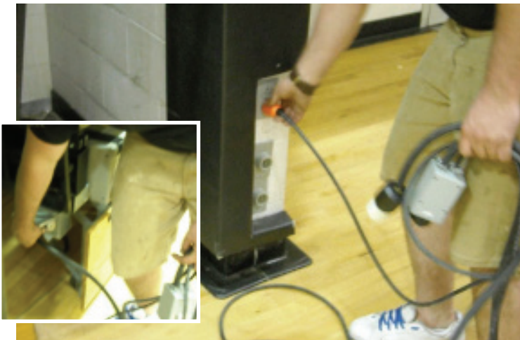
Pendant controls must be plugged in to the power supply and the bleachers (inset), to operate bleachers.
