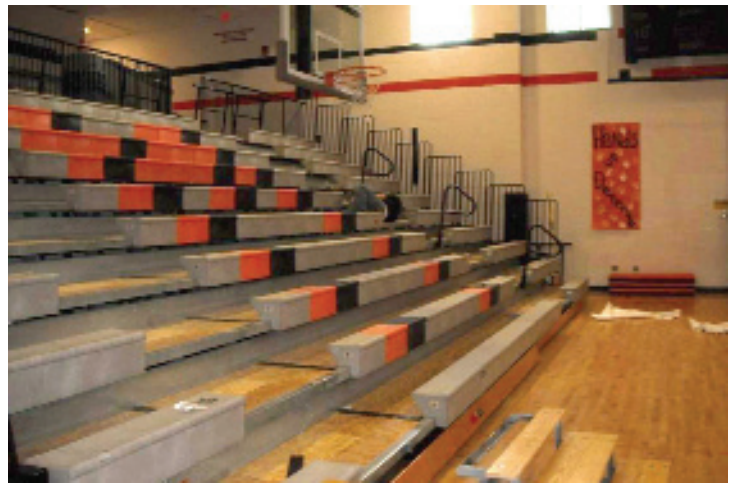
Bottom-line savings compared to buying new -- in excess of 50%. Owners representative was King & King Architects.
