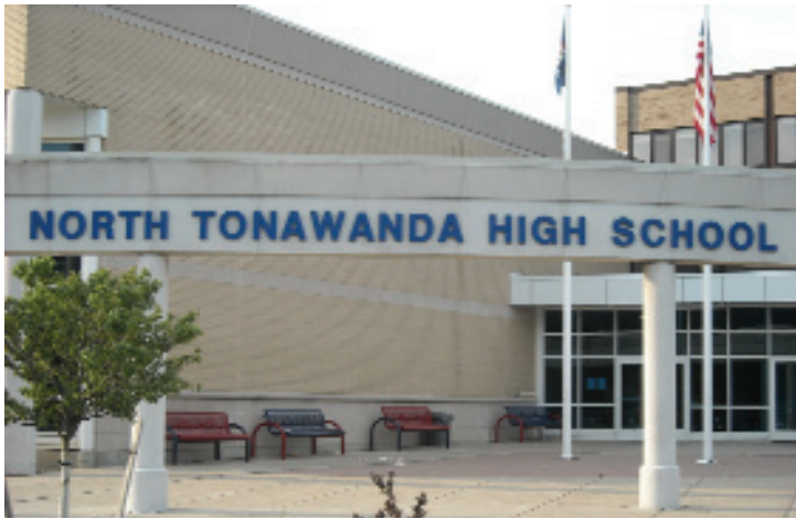
North Tonawanda High School is near Buffalo, NY. This was a 3-gym project, the first project was the “old gym.”
