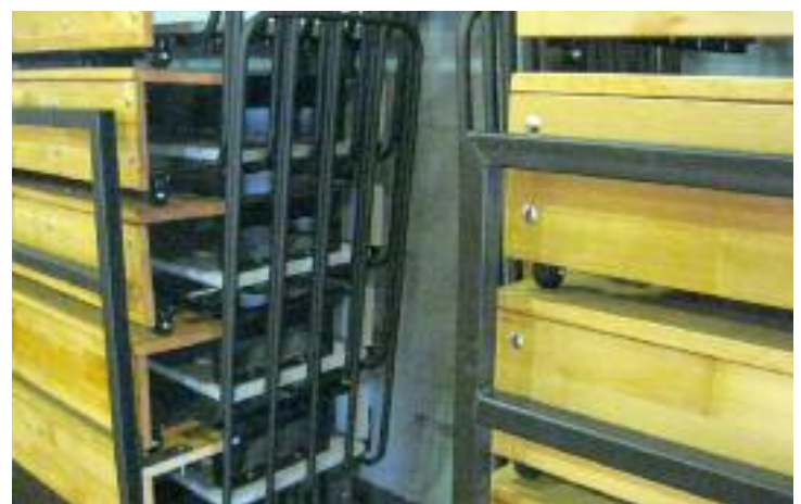
Showing end safety rails and Century Design® system at end of bleachers.
