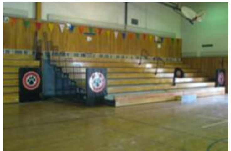
Photo shows one bank in open position. Note demountable first row step at aisleway. All intermediate steps have non-skid tape.
