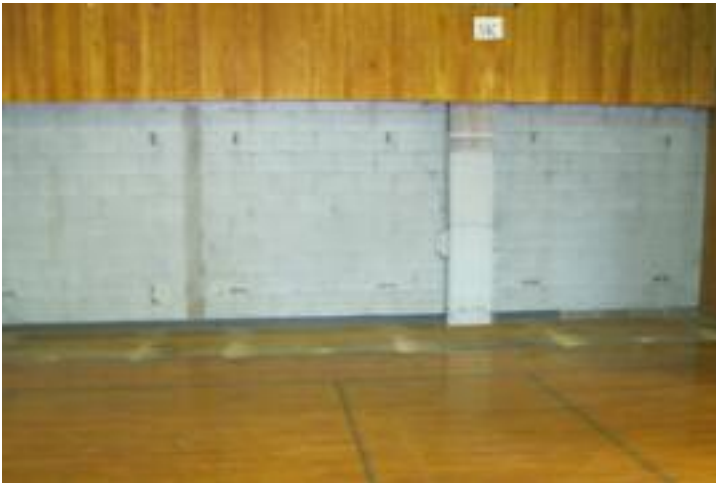
Removal down to bare walls is complete.
