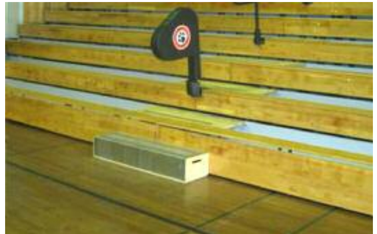
Photo shows seat-level aisles with demountable first row step. In addition to providing better ingress/egress, these aisles provide support for the Century Design® system that is installed at the aisles.
