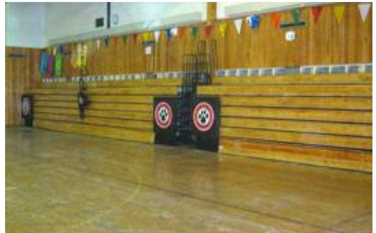
Removable padding for both ADA rails and P-rails is seen in this photo.
