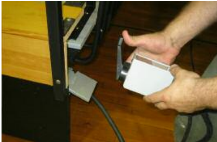
Removable pendant controls for motorized drive are a safety feature -- only authorized maintenance personnel can open and close the bleachers.
