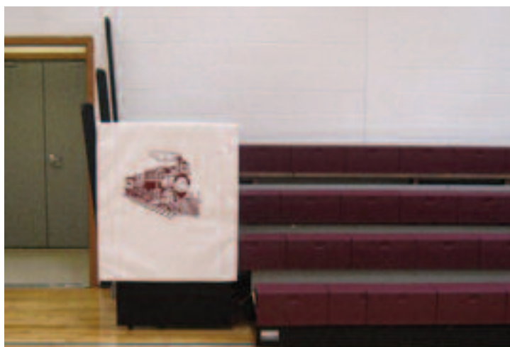
On the "visitors" side of the gym, the bleachers are four rows high. This photo shows ADA cutout at end of bleachers, with padding on safety rail. Note end safety rails at the end of rows 2, 3 and 4.
