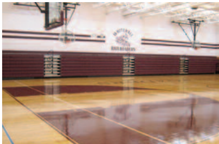
Wide angle photo shows completed job with new plastic seat modules in school colors, self-storing P-rails at aisles. Note newly refinished gym floor, basketball backstops, lights, etc.
