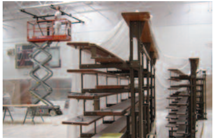
Photo shows bleacher understructures before they were removed from gym and stored, so that gym refurbishment work could continue without the bleachers being in the way.
