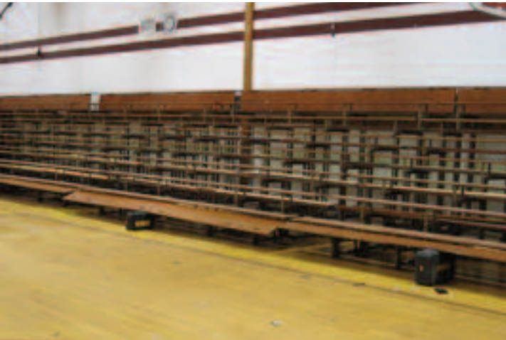
Most of the boards have been removed in this picture. Lumber was recycled for use as footboards and heelboards in the new "closed deck" bleachers.
