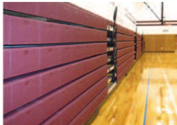
Straight, even row spacing shows these bleachers are not sagging. With the Century Design® system in place, these bleachers will not sag.
