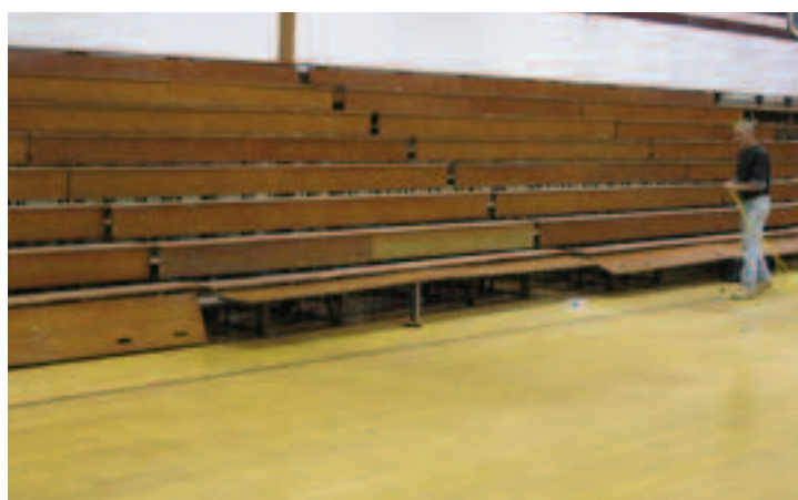
Bleacherman crew member begins to dismantle the original bleachers.
