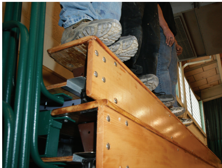
The Century Design® system allows for climbing or loads in the closed position (unintended for occupancy).
