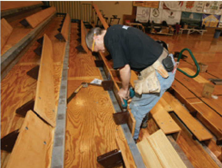
Attaching the mounting hardware for seats and risers.
