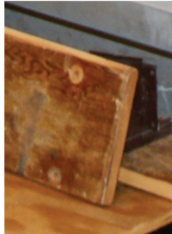
At left: 50-year-old douglas Fir boards were showing their age when removed for refinishing. At right: after being planed, sanded and edged, the refinished lumber was reinstalled with new hardware.
