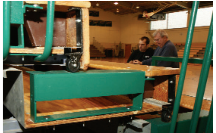
Century Design® system is installed on ends to provide continuous support in any configuration. Bleachers can't sag, because the wheel mounted on the row above rides on the rail and seat below. Safety rail temporarily removed to show Century design detail.
