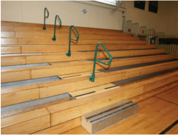
Photo shows aisles with P-rails, first row step and non-skid tape.
