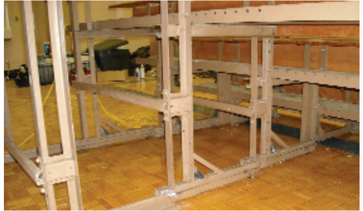
The understructure was thoroughly cleaned and repaired.
