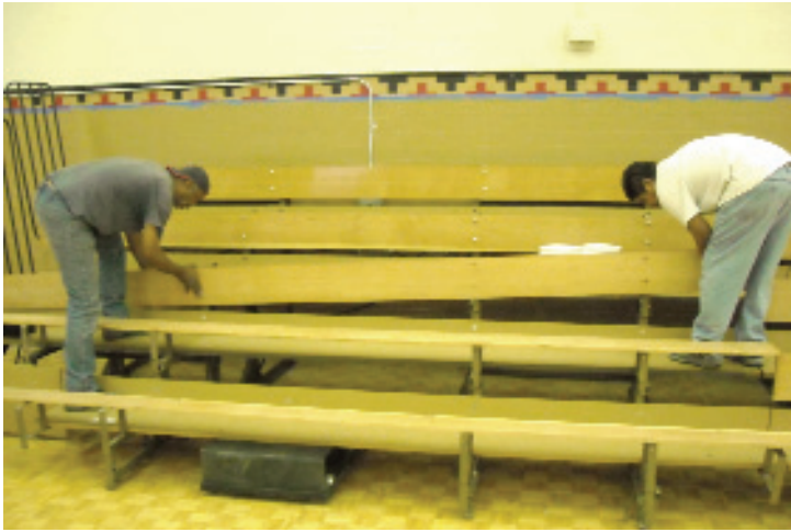
After refinishing, boards are reinstalled.
