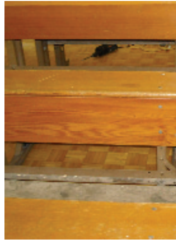
At left: Open deck of original bleachers. At right: new heel-board and partial footboard (seen here with a primer coat of white) now make this a closed deck. Bleachers are safer, because a child's foot cannot pass through the opening.
