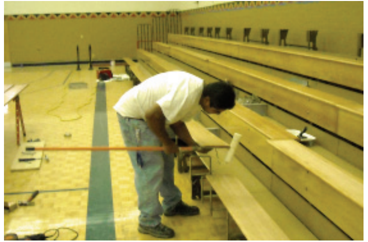
Photo shows employee refinishing seats with three coats of approved sealer.
