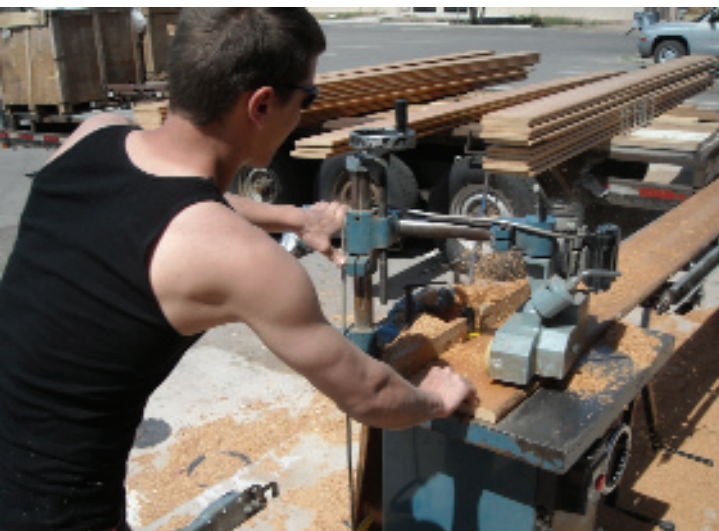
Boards were planed, edged and sanded outside, to minimize the mess.
