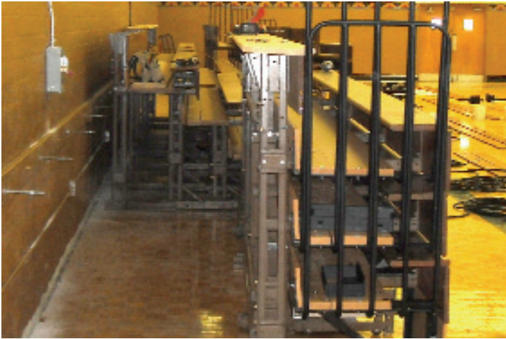
Bleachers on both sides of the Community Center were unanchored from the wall and moved to make room for cleaning and refinishing.
