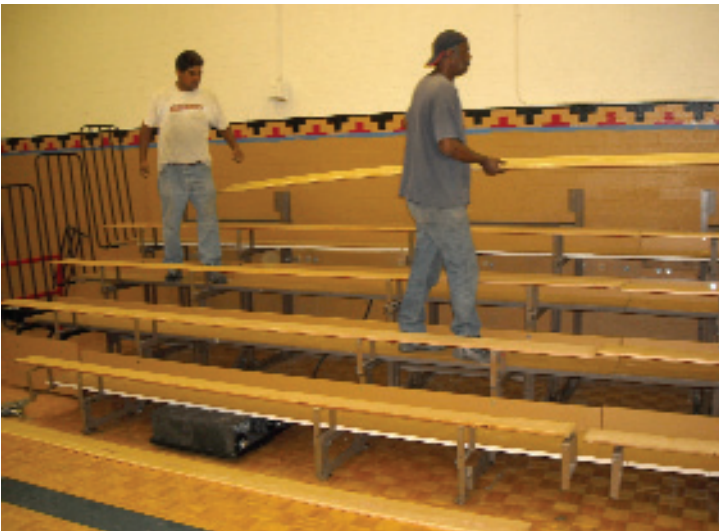
Seats and risers being removed for refinishing.
