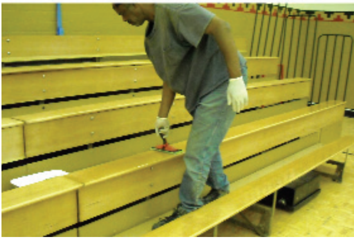
Seats are topped off with a high build clear coat sealer.
