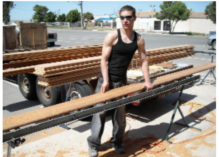
All removed lumber was taken outside for refinishing.
