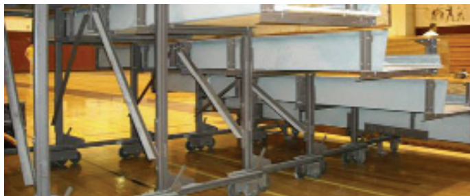
Close up of bleacher section in the open position.
